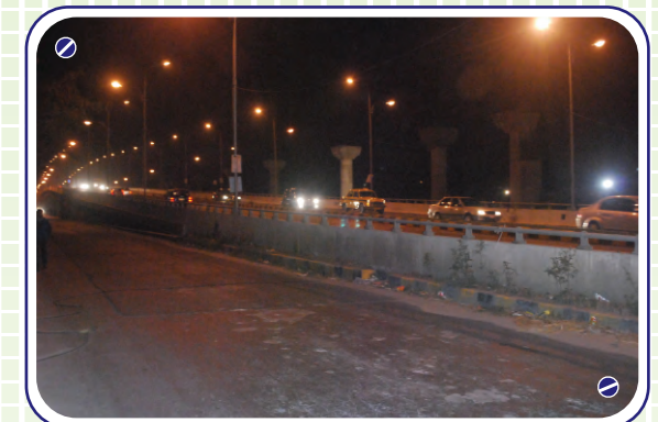
Night View of the flyover at Action Area I, New Town
